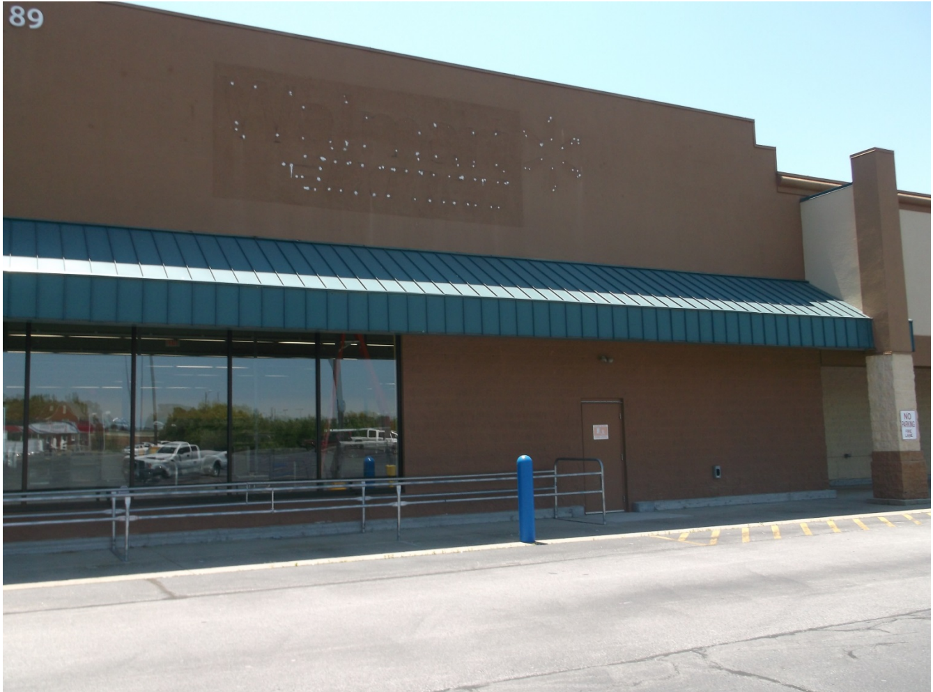
Photo #5 – Exterior view of the brick veneer and metal stud framing behind the storefront.
