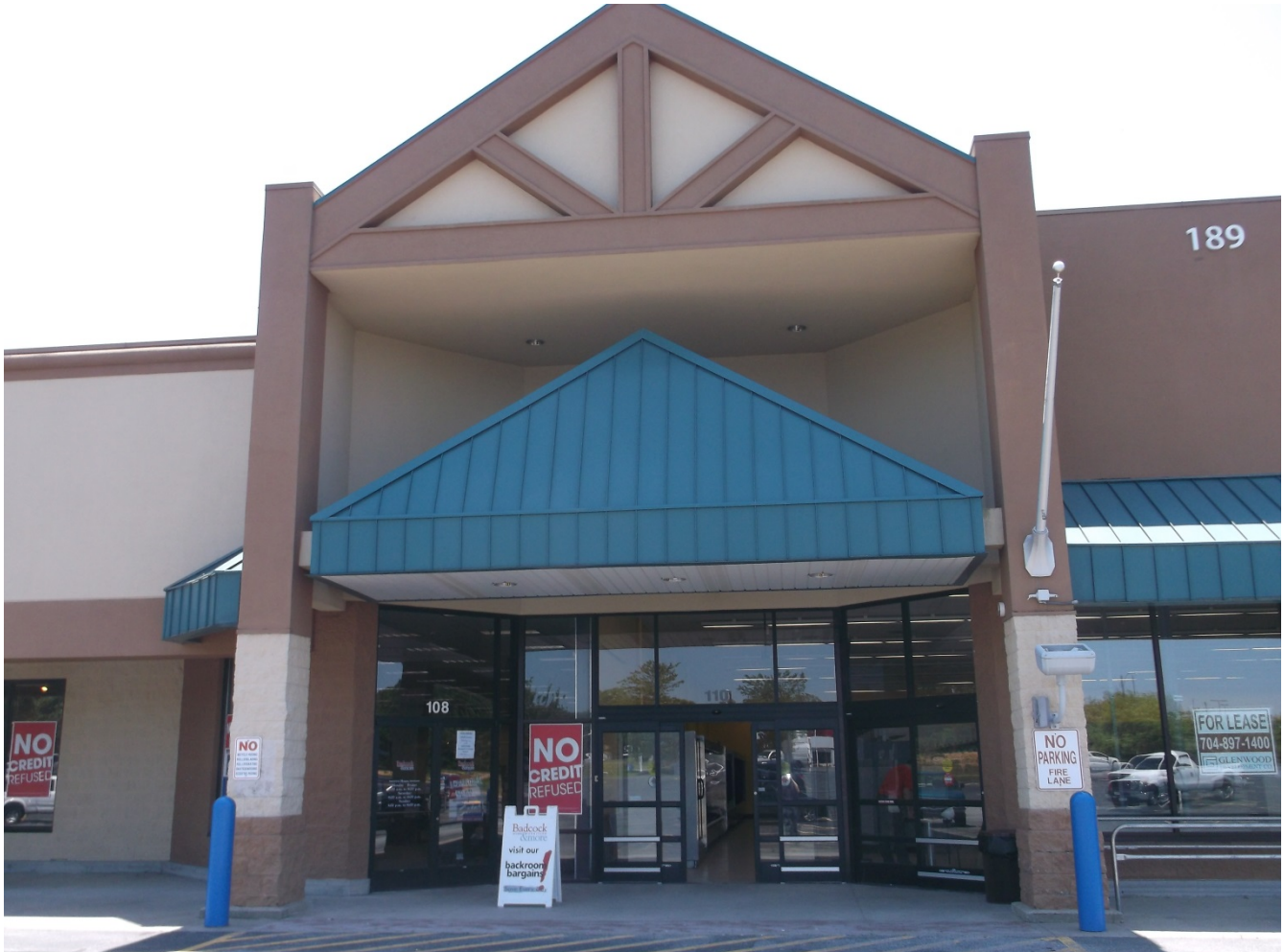
Photo #1 – Former Walmart Express – exterior of front of building. The unit is next to Bedcock Furniture in a Marketplace in Winston-Salem, NC. There are three structural steel columns and splitface CMU wraps at the front of the building.
