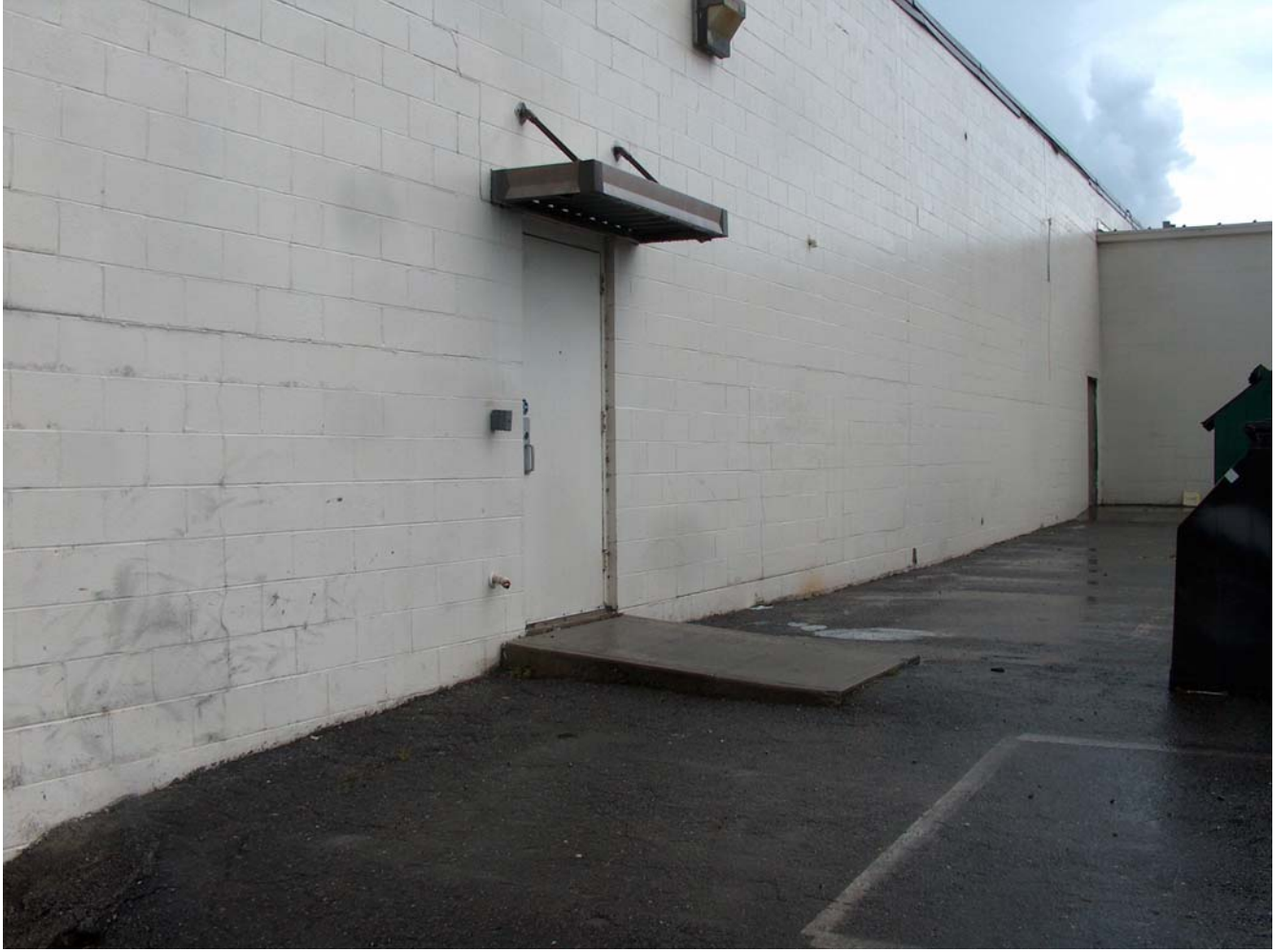
Photo #6 – Egress door leading out from stockroom with concrete slab. Concrete slab is raised up from surrounding asphalt – typical for both exterior doors on this side of the building.
