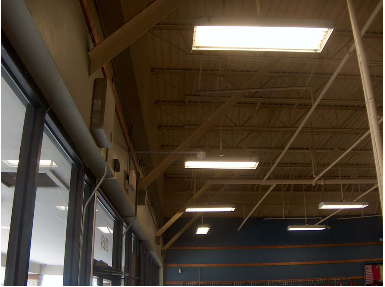
Photo #12 – Steel L3X3 braces extending up from lintel beam over storefront to roof structure above. The angles may be exposed if Dollar Tree provides a new ceiling.
