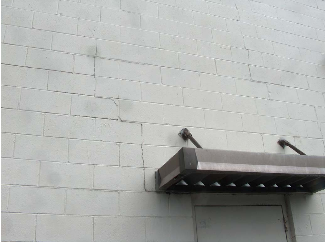
Photo #8 – Cracking of CMU side wall above personnel door – typical for both doors.
