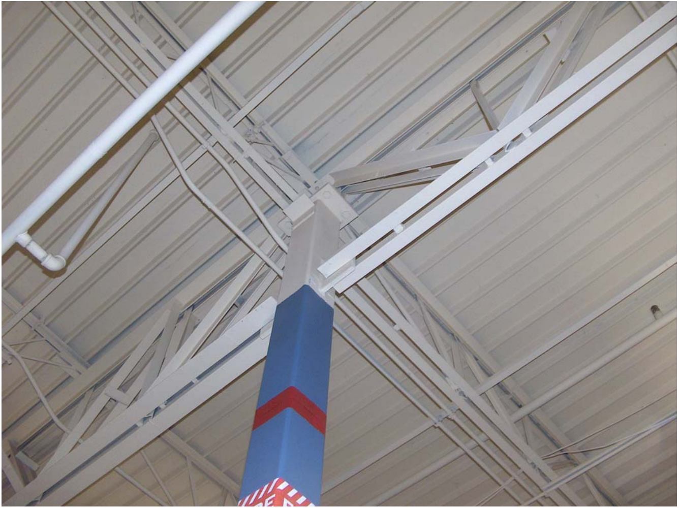
Photo #2 – Interior HSS6X6 steel column supporting 32” deep joist girders, steel bar joists and metal decking. There is no ceiling located within the proposed Dollar Tree space.
