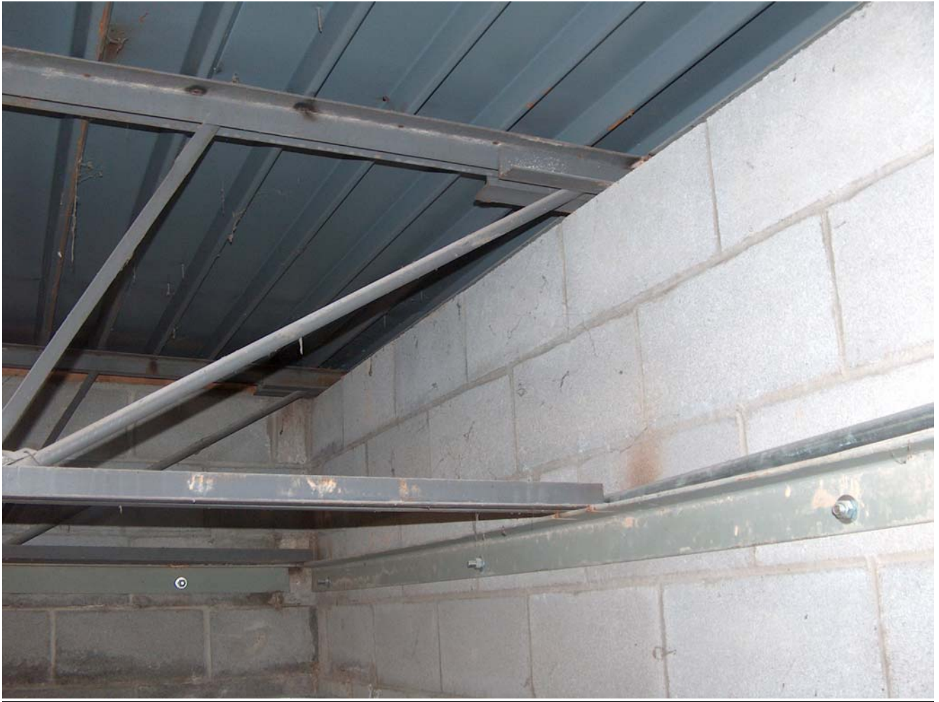
Photo #3 – Rear exterior 12" CMU load bearing wall with 22" deep joist bearing on top of wall.
