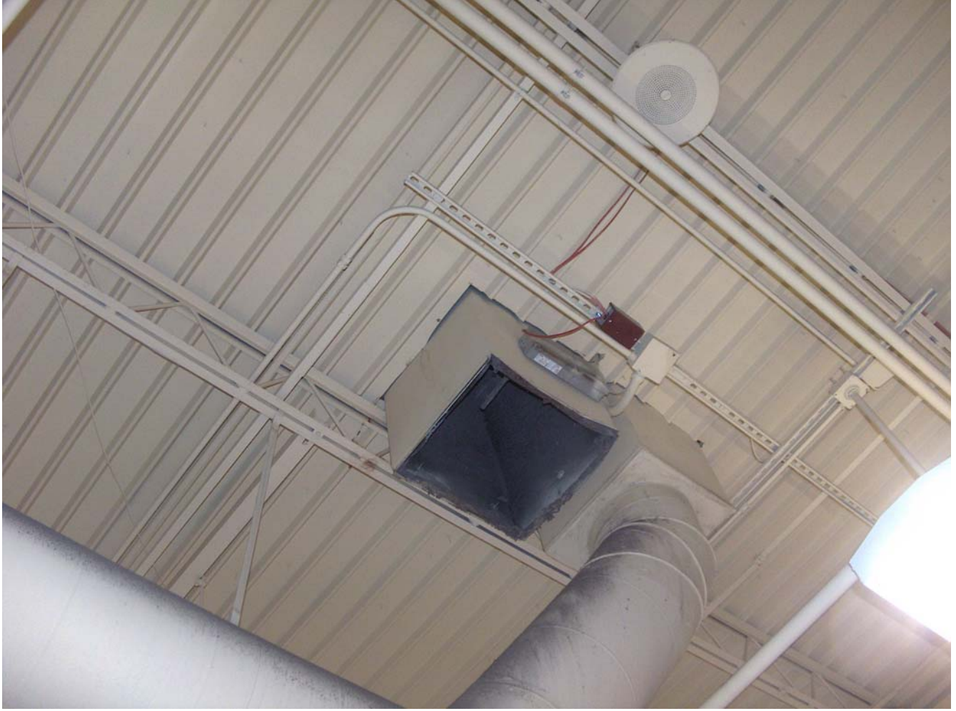
Photo #11 – Rear Trane RTU with no support below existing curb.
