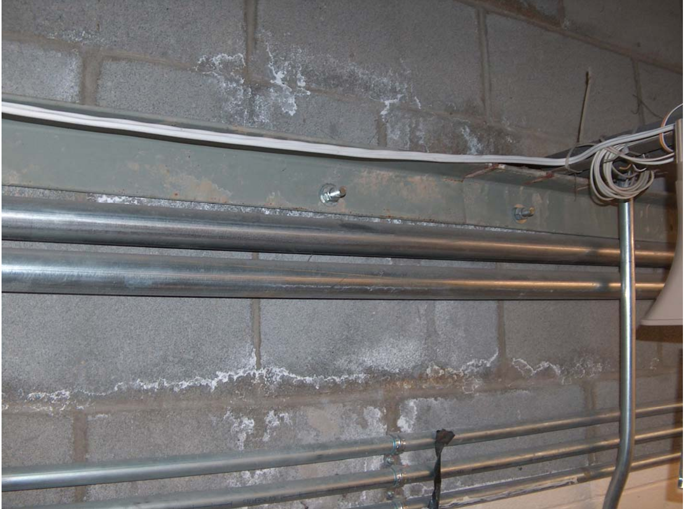
Photo #9 – Efflorescence located on inside face of CMU rear bearing wall. Water has been getting inside wall cavity.
