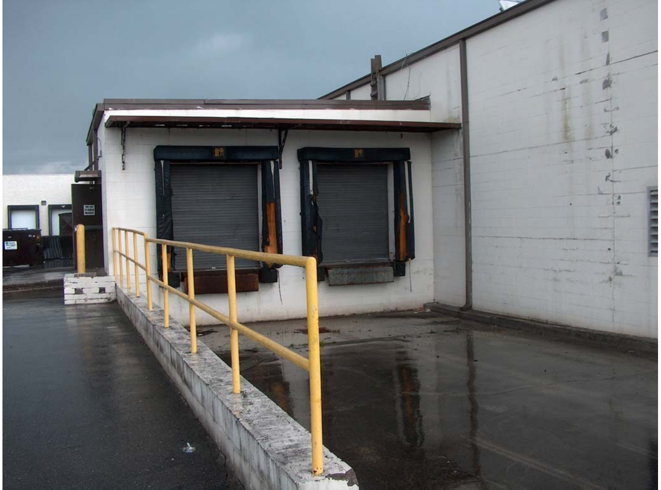
Photo #5 – Recessed truck ramp and loading dock. Dollar Tree would have loading dock closes to exterior wall.
