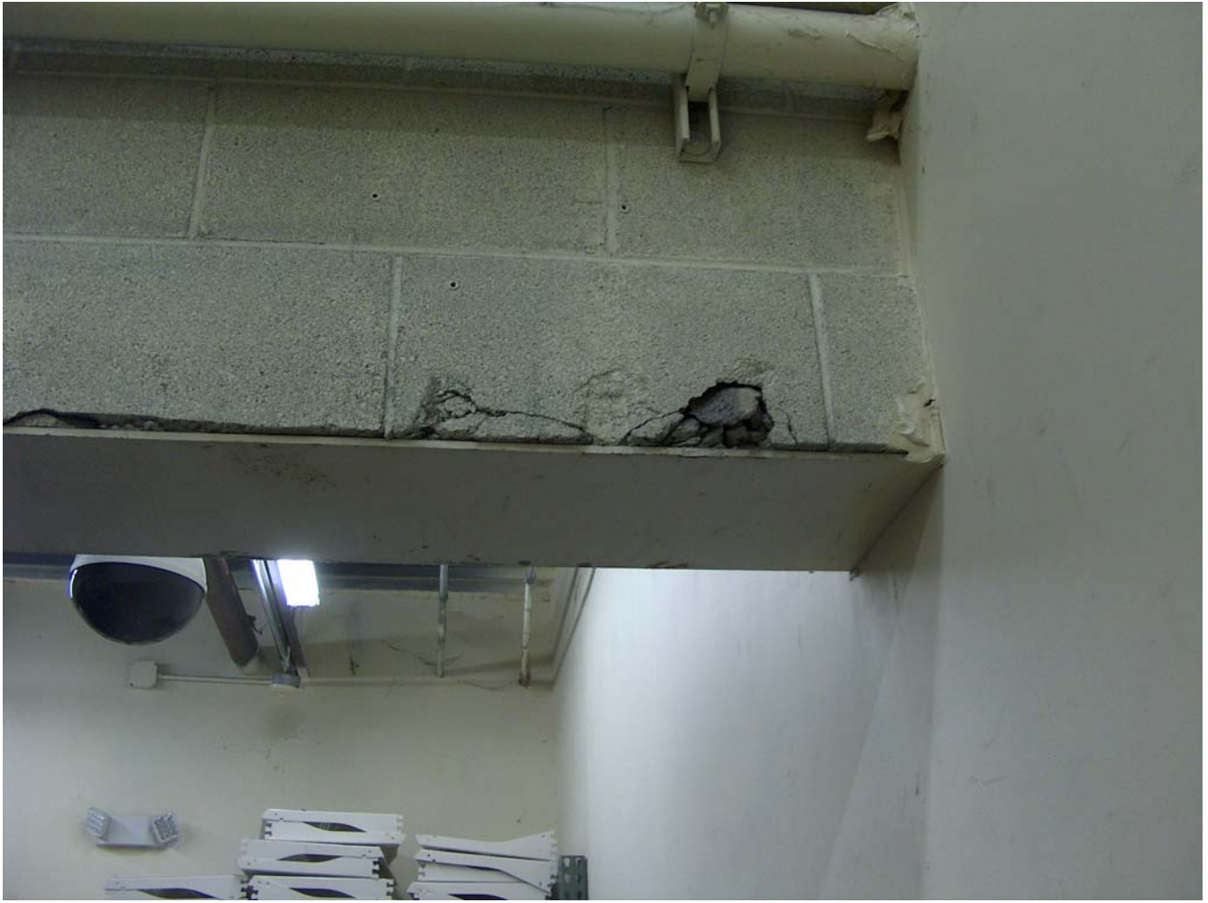
Photo #13 – Cracked CMU face shell above steel lintel plate around the rear stockroom entrance. We recommend that the broken CMU be replaced with grout to maintain bearing.
