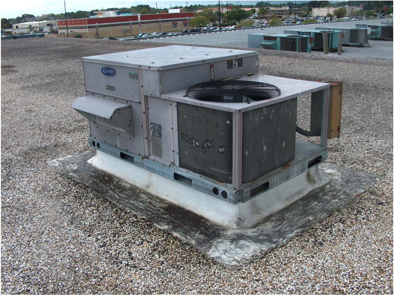
Photo #10 – Existing Carrier RTU located over proposed Dollar Tree space. There are 7 units total – a combination of Trane and Carrier. This unit appears to be in an original location.
