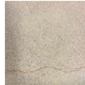
stained polished concrete
